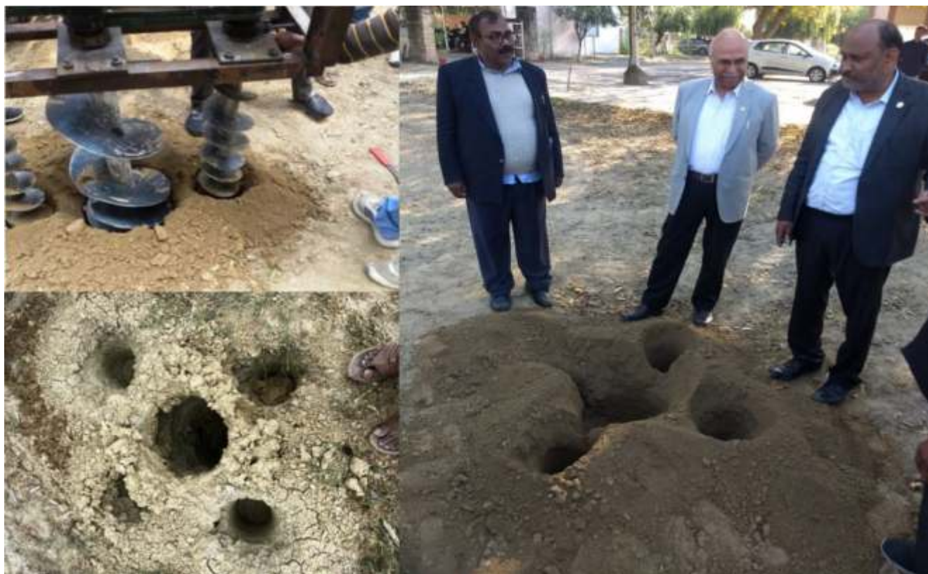
Fig. 5.9 Process of making auger hole in sodic soil.
